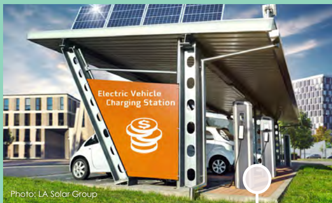
Solar PV canopy integrated with EV charging on open parking area
