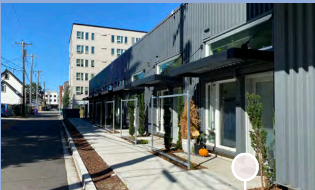
Simple screening design can be easily altered to meet future needs
