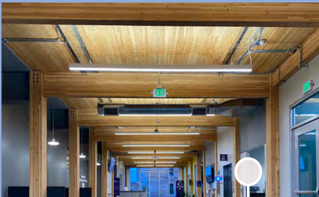
Mass timber construction
