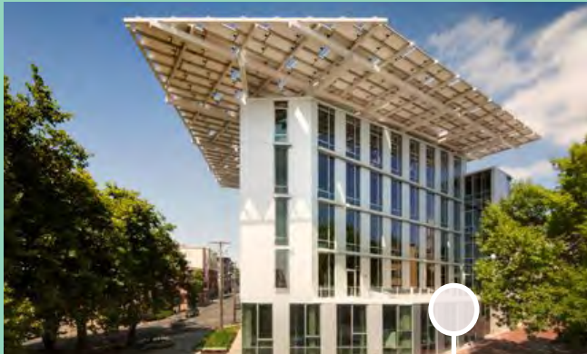
Photovoltaic roof array also provides shade from heat of summer sun
