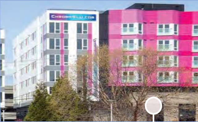
Colored bays and white “bar” on left make distinct parts of larger building
