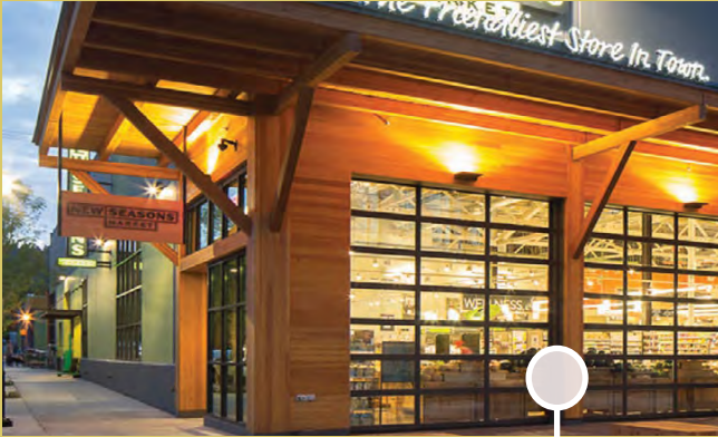
Exterior accent lighting
