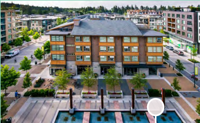
Hardscape plaza can support overflow parking at major events
