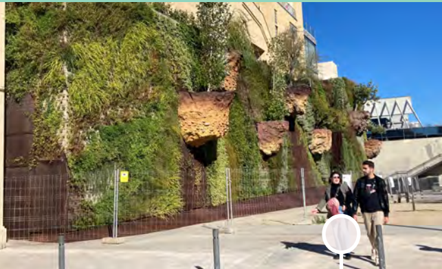
Structural pockets in vertical green wall
